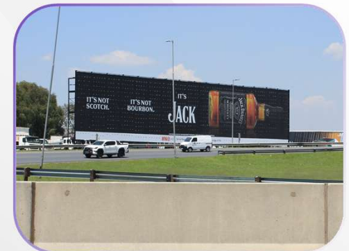
Reitfontein Mega Hoarding
